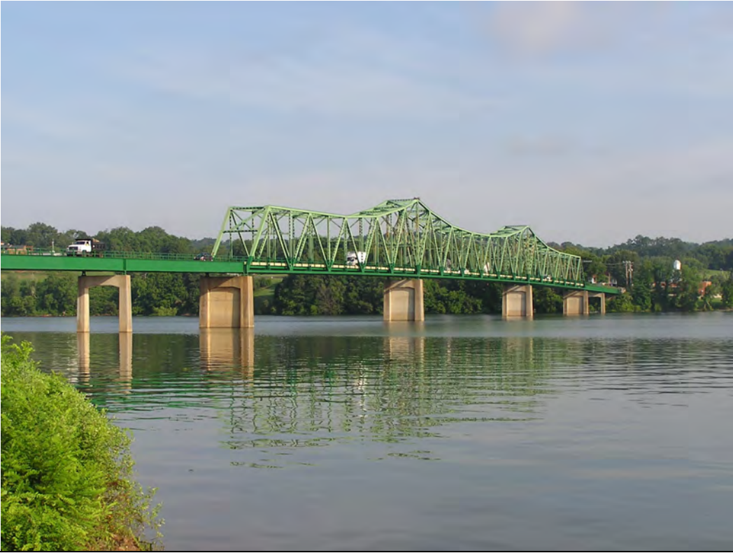
Photo 1: View of SR-92 bridge over French Broad River facing northwest.
