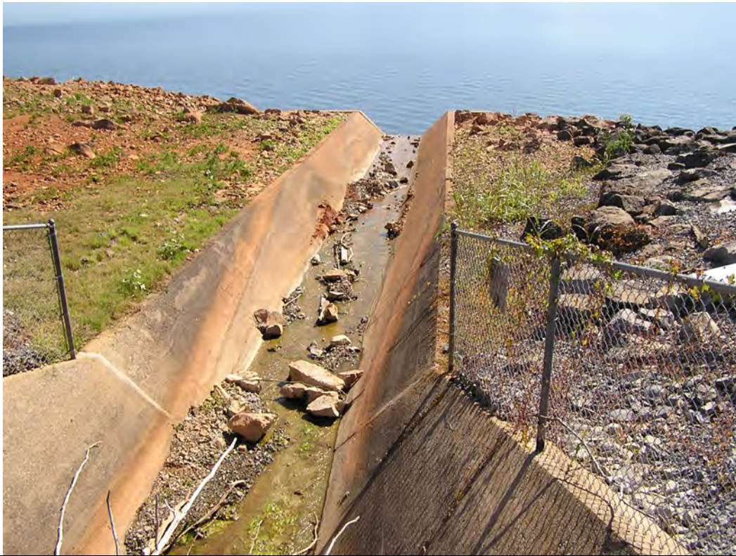
Photo 7: View of STR-2 facing southeast.
