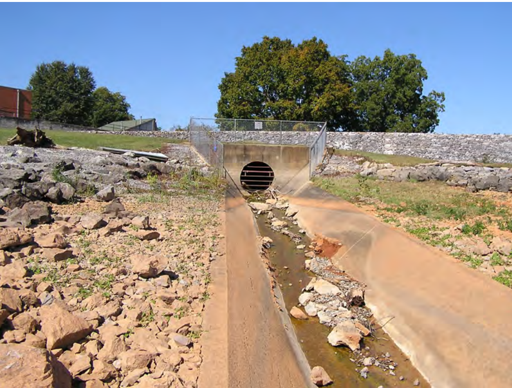
Photo 8: View of STR-2 facing northwest.
