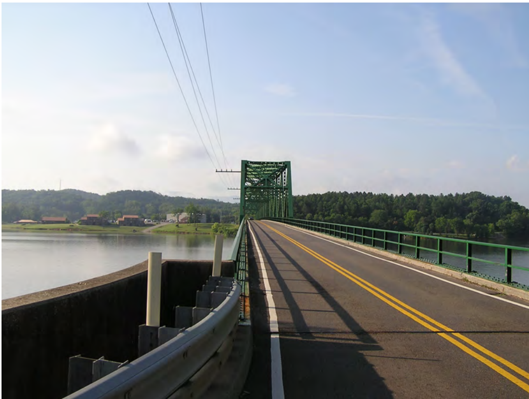
Photo 4: View of SR-92 bridge over French Broad River facing southeast.
